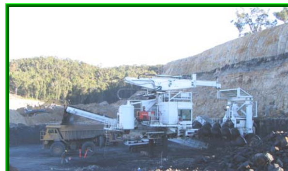
Auger operating in elevated position and direct loading trucks
